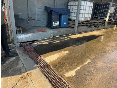
Existing Drainage around washbay
