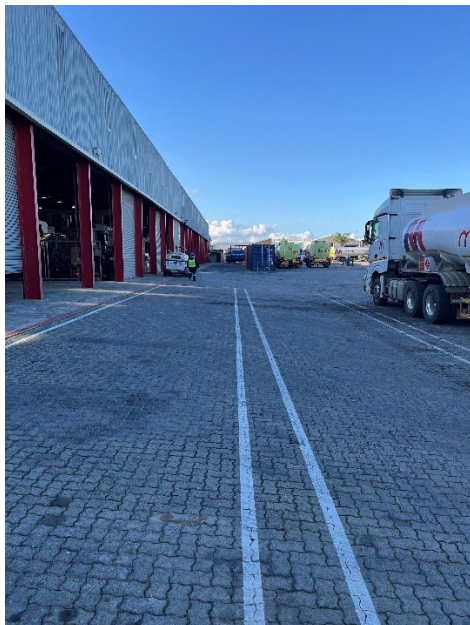
Gutters on existing buildings
