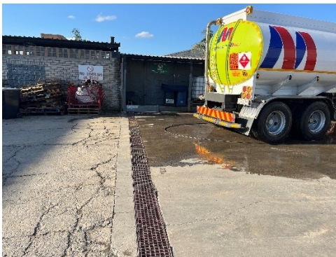
Existing Drainage around washbay
