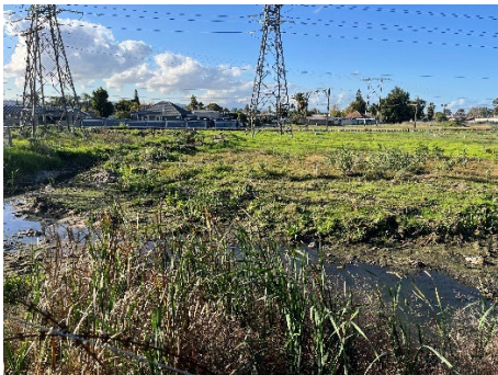
Pond to west of site into which stormwater discharges
