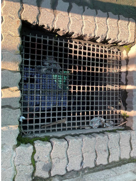
Existing stormwater inlet on western boundary
