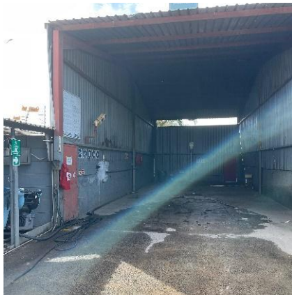
Figure 6.4. Site Image: View of the internal building (wash bay) to be demolished.
