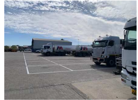
Figure 6.12. Site Image: View of the truck parking area.
