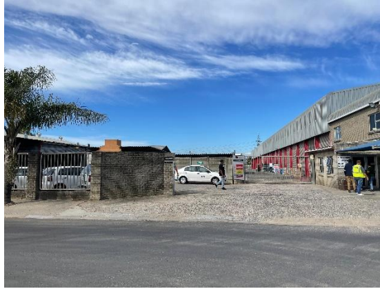
Figure 6.2. Site Image: View of existing entrance/exit gate.
