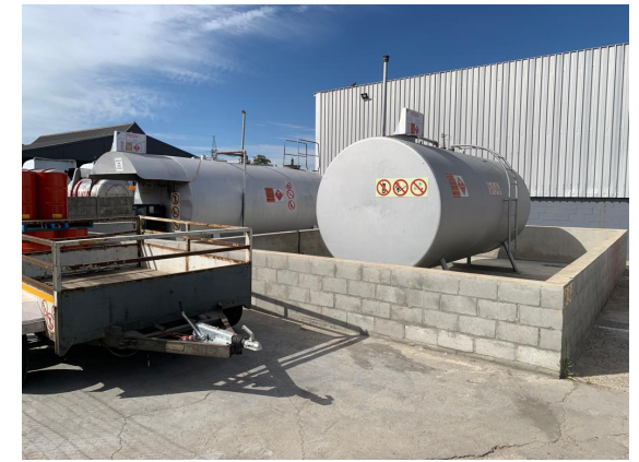
Figure 6.6. Site Image: View of the two existing tanks housed within a bund.
