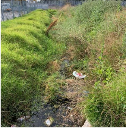
Figure 6.19. Site Image: View of water pollution in the channel.
