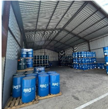
Figure 6.11. Site Image: View of oil drum storage structure to be demolished.
