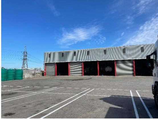
Figure 6.13. Site Image: View of workshop.
