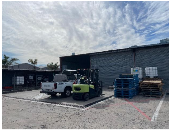
Figure 6.5. Site Image: View of the building extending from wash bay to be demolished.
