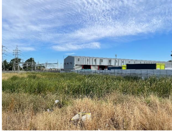
Figure 6.14. Site Images: View of the western boundary of the project site.
