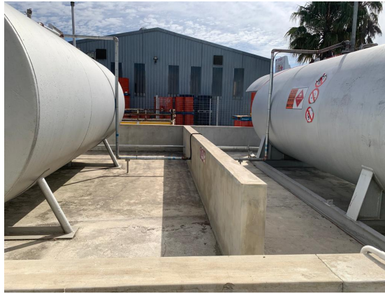
Figure 6.8. Site Image: View of the intermediate wall between the tanks housed in a bund.
