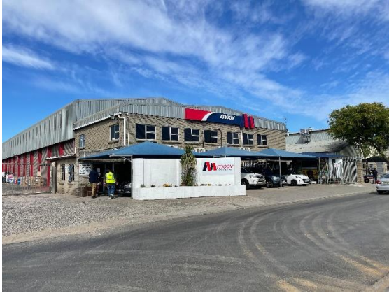
Figure 6.1. Site Image: View of entrance building from Kiaat Road.
