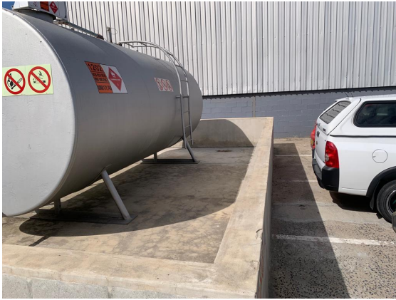
Figure 6.7. Site Image: A closer view of the tank bund wall and floor.
