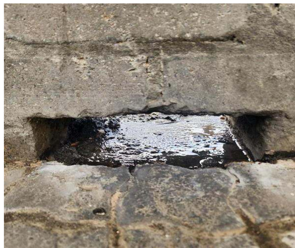
Stormwater outside admin building
