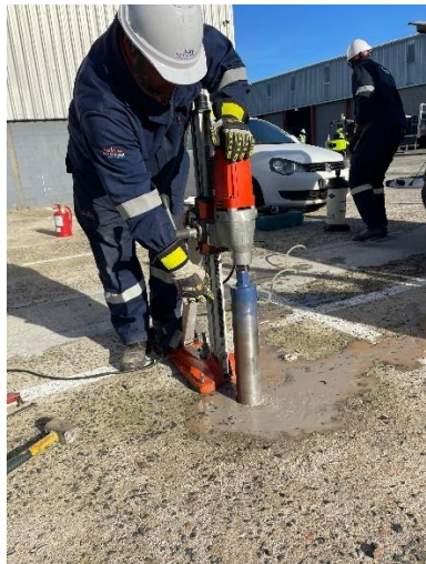
PHOTO 3: Core drilling to break through concrete surfacing.
