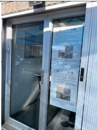
Photo 3: Notice pair 2 placed on a secondary entrance door to the project site.
