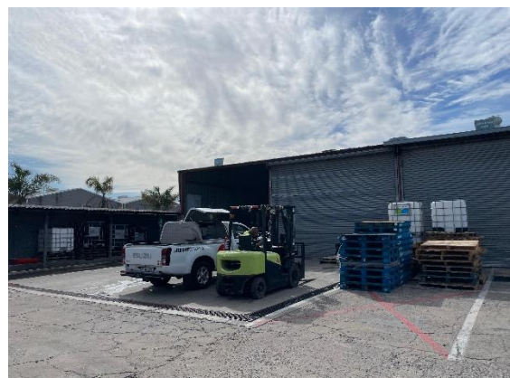
PHOTO 5: View of building extending from wash bay to be demolished.
