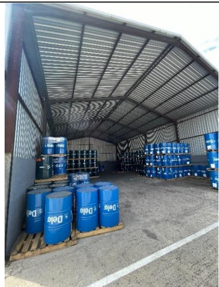
PHOTO 11: View of oil drum storage structure to be demolished.
