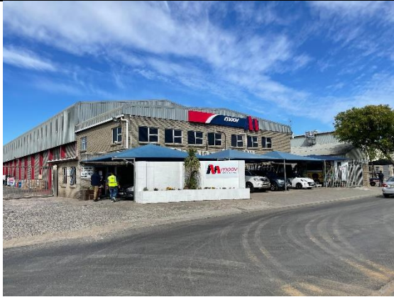
PHOTO 1: View of entrance building from Kiaat Road.
