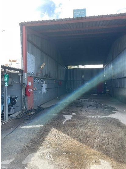
PHOTO 4: View of internal building (wash bay) to be demolished.
