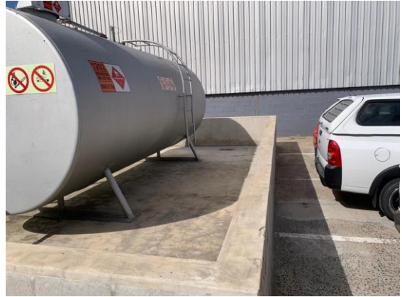
PHOTO 7: Closer view of the tank bund wall and floor.
